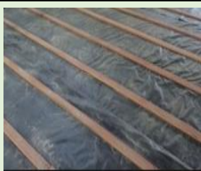
Plastic Membrane Install plastic/battens
