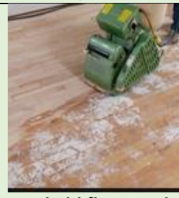
Sand old floor to clean Fix sub Floor
